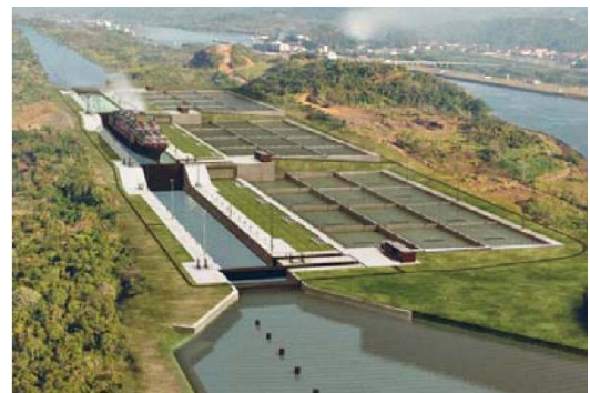
Fig.2 Conceptual view of the expanded Panama Canal locks with “side ponds” (Image from Internet)
