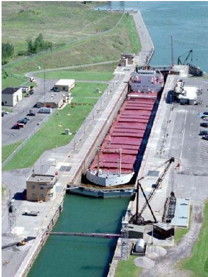
Fig.1 The Eisenhower Locks in Massena, New York (a “simple” lock) (Image from Internet)
